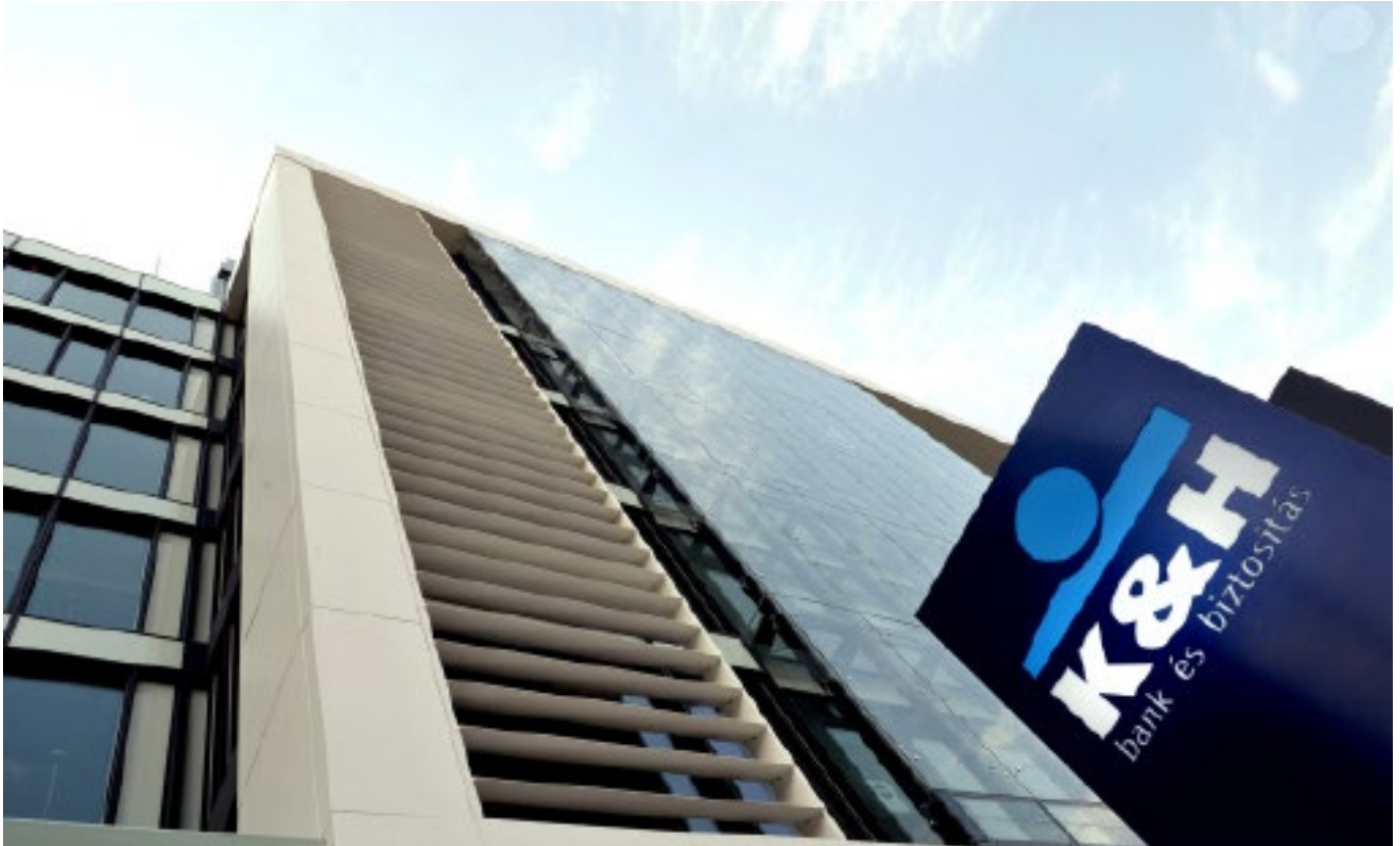
K&H's head office building in Hungary.
